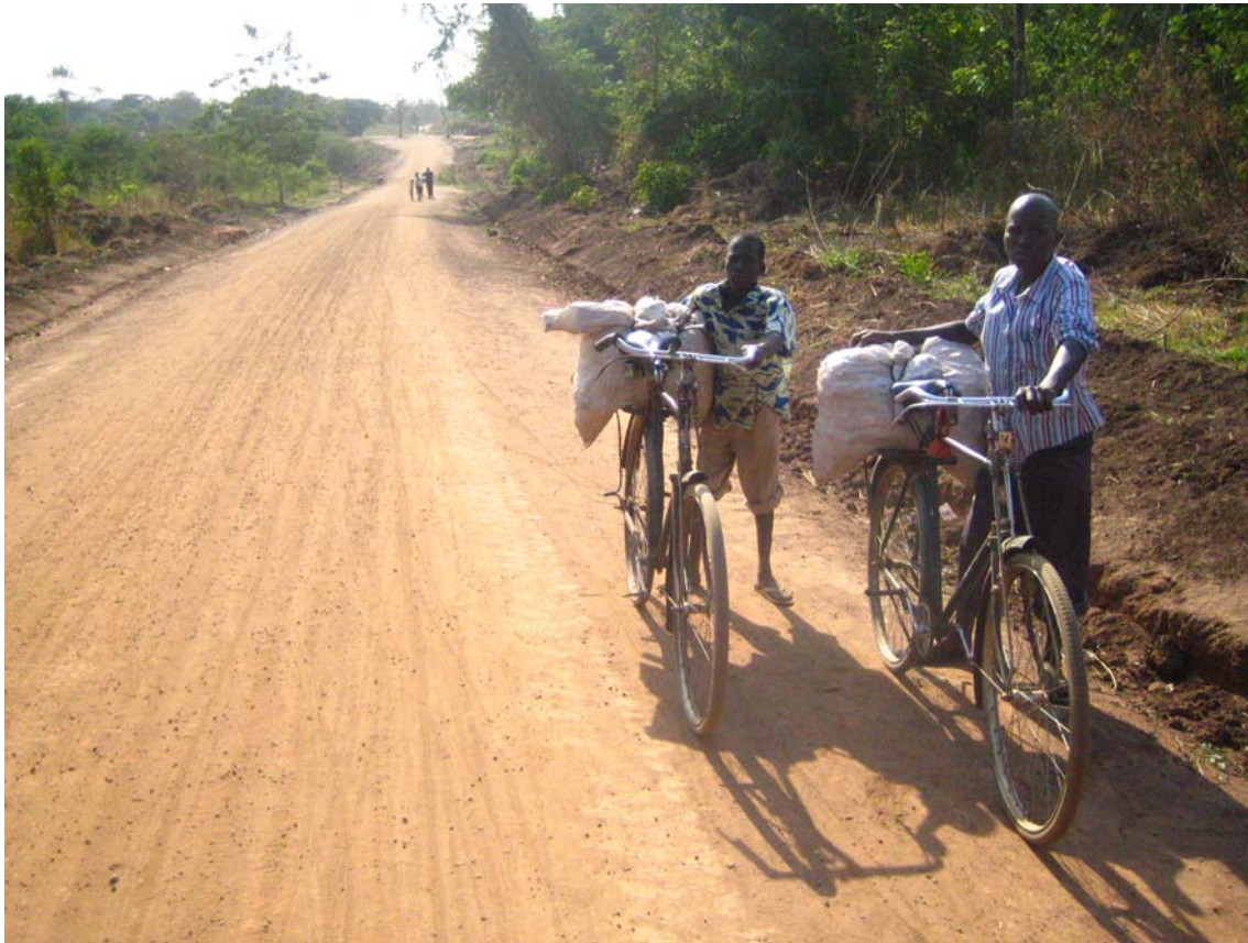
Beneficiaries using a newly graded community road
