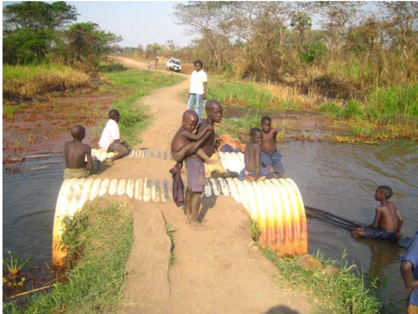
A community road before construction
